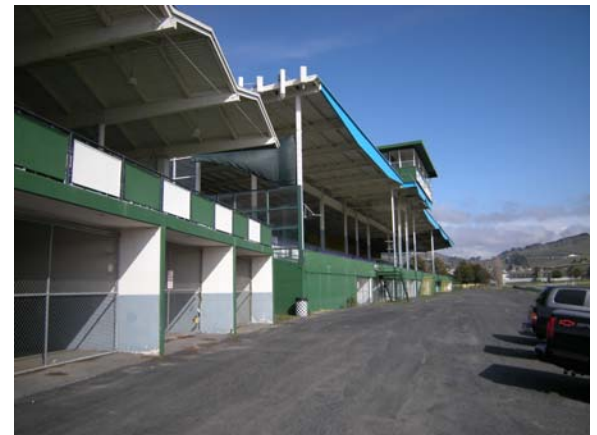
View of Grandstand looking North (Constructed of concrete, wood & steel) Lack of lateral bracing at roof support
