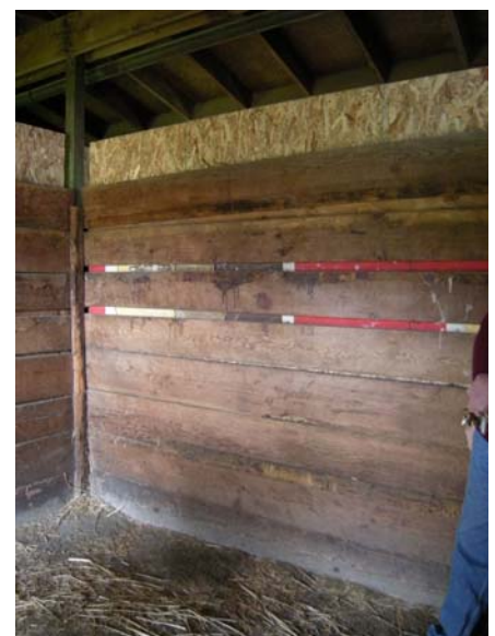
Typical Stall w/ sheathing added.
