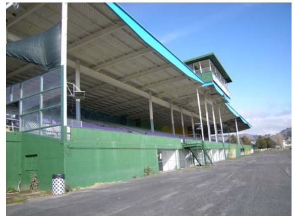
Existing Press Box and Structural Support of Roof w/ no lateral bracing
