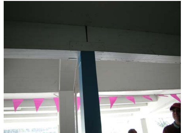
Beam Support at Column at Grandstand Splaying connection. No lateral bracing.
