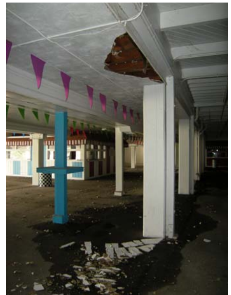
Roof Leaks & Deterioration @ Grandstand (Concrete & Wood Construction)
