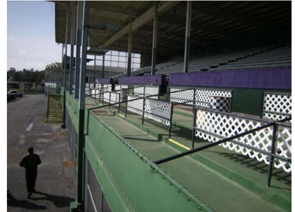
Accessibility Issues and lack of structural bracing.
