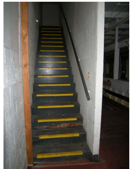
Grandstand Stairs to Press Box Lack of landing and extended handrails
