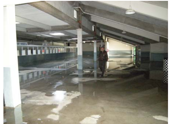
Water Infiltration at Grandstand
