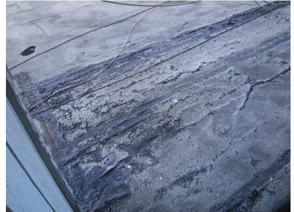
Deteriorated Roof at Grandstand (close-up)
