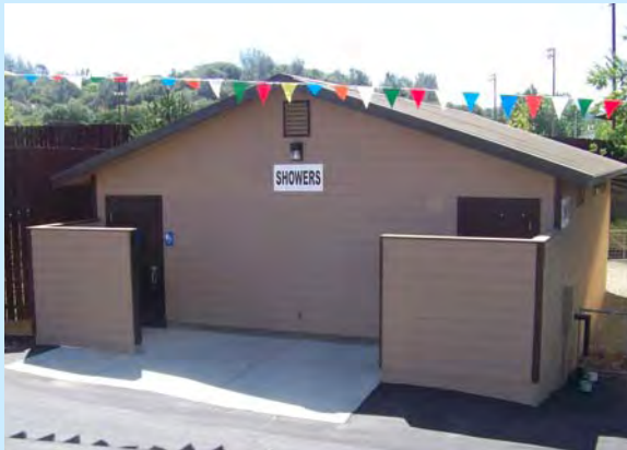
A new restroom with showers at the Mariposa County Fairgrounds. Shower facilities are an important feature for fairs being utilized as emergency staging areas.
